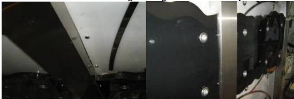
Picture 34 the ceiling cladding with acrylic and stainless steel
