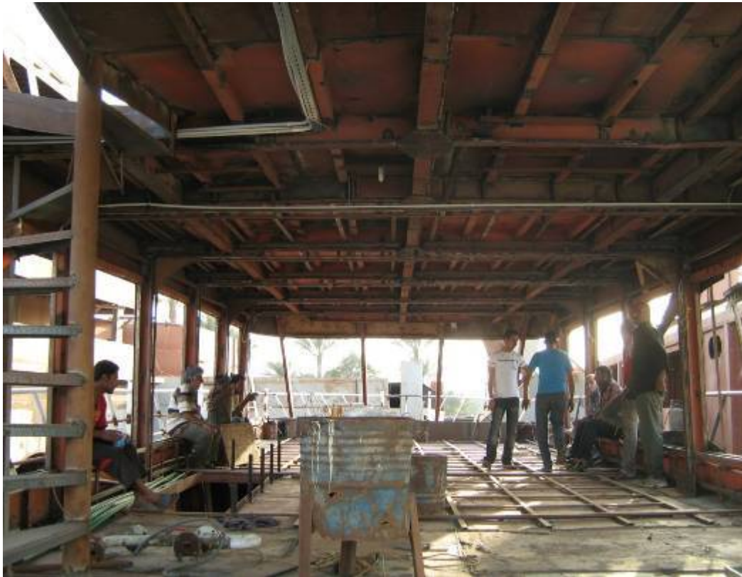
Picture 28 implementation of design were started with fixing a iron structure
